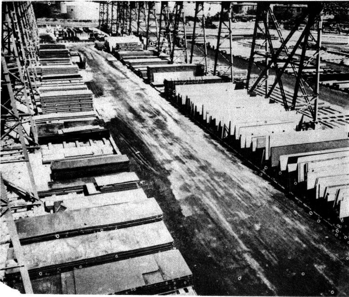
Figure 5-52. Storage of heavy plate and structural shapes.
